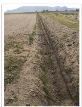
Installing Drip Irrigation
