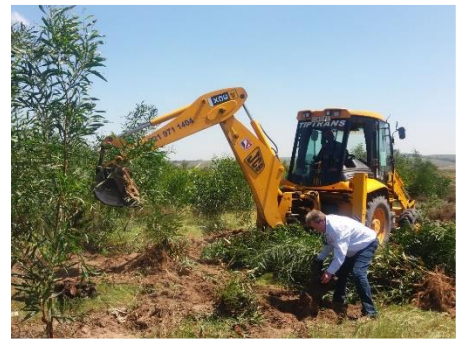
Clearing land & planting preparation
